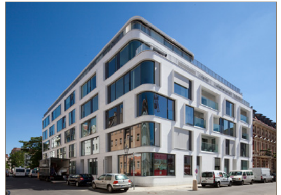
The building should be shown in full
